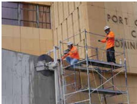
*Workers from Concrete Coring Company with the special saw designed to cut the tile from the wall.*
